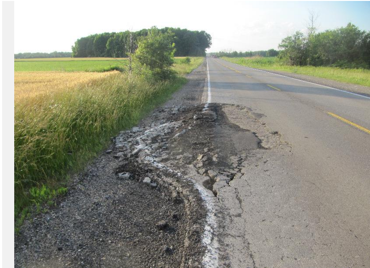
At least half of the highway lane is encompassed by a road surface failure on Wonderland Road yet no warning is provided of its existence.
