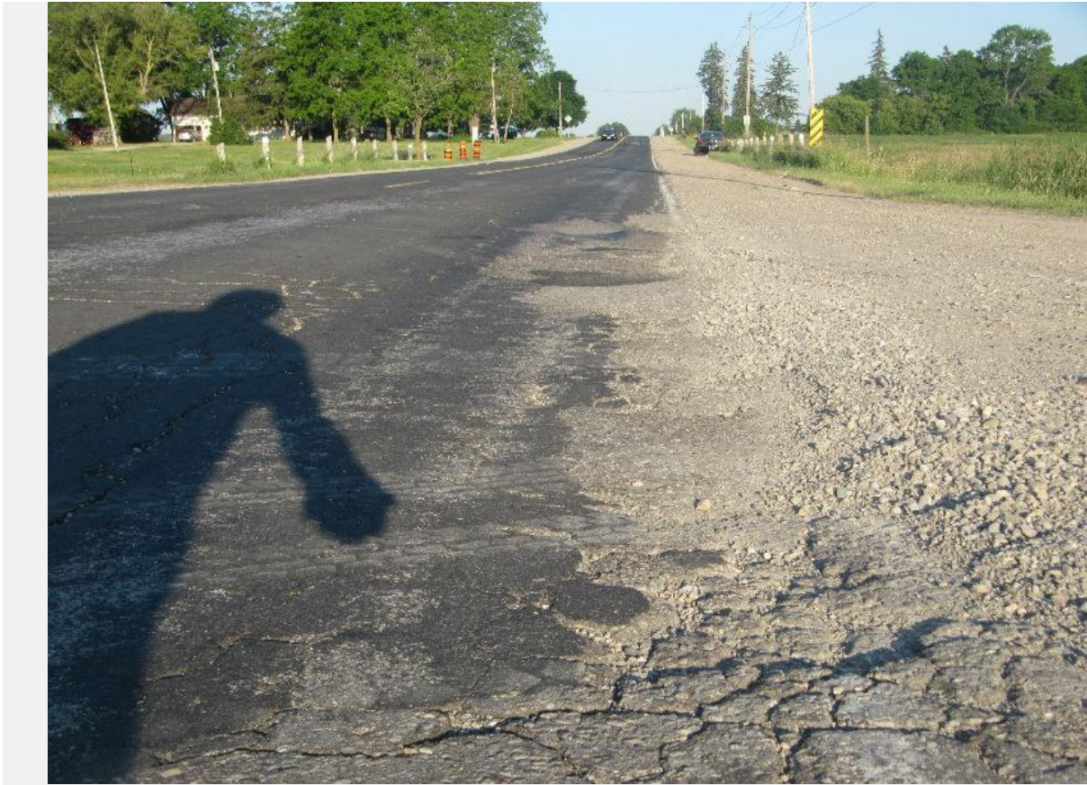
View of the broken and deteriorated pavement of the westbound lane of Wilton Grove Road at a location just east of the point of impact.
